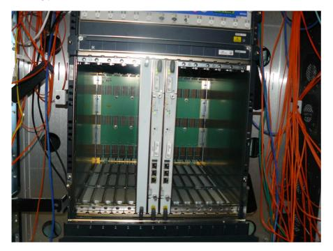
Figure 9. T1600 with Routing Engine
