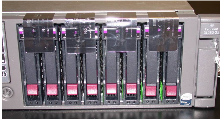
Figure 4: Tamper Seals over Front Hard Drives
